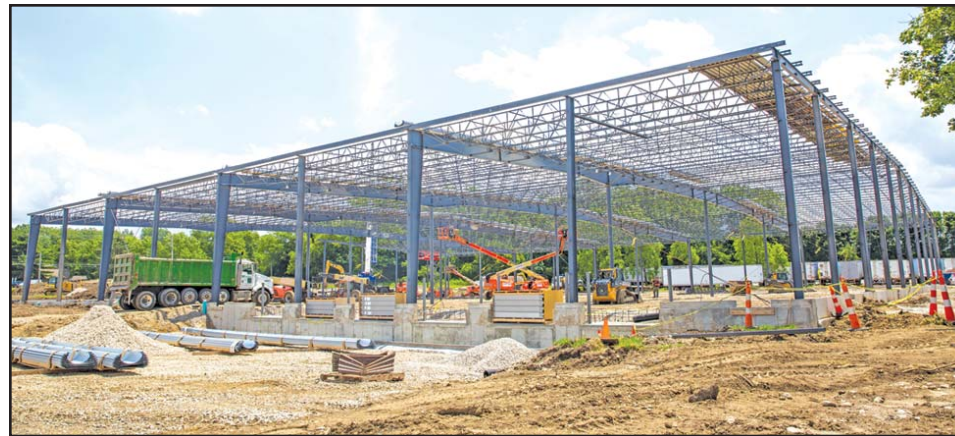
In-progress construction of American Excelsior's new facility in Norwalk
