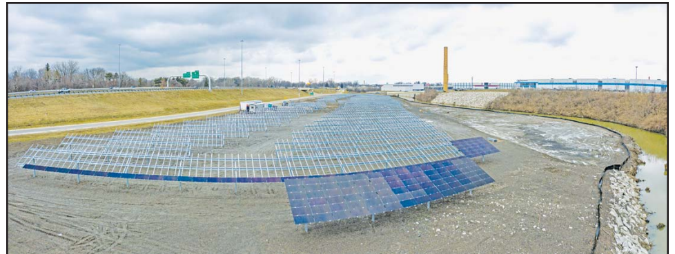
Previous progress on the solar array in Overland Industrial Park
