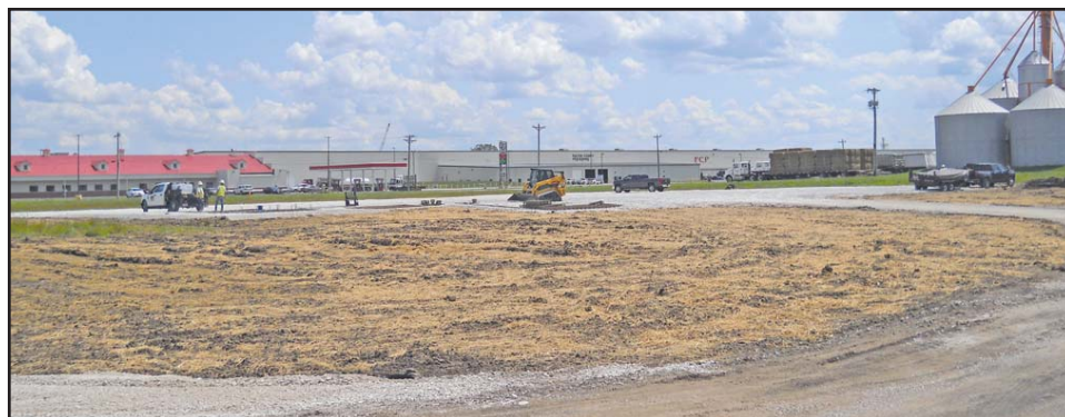
The site for the new electric distribution substation in Fulton County
