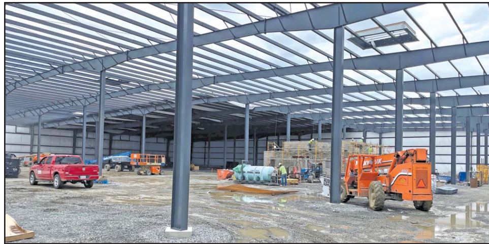
Interior construction on Randall Bearings' new facility
